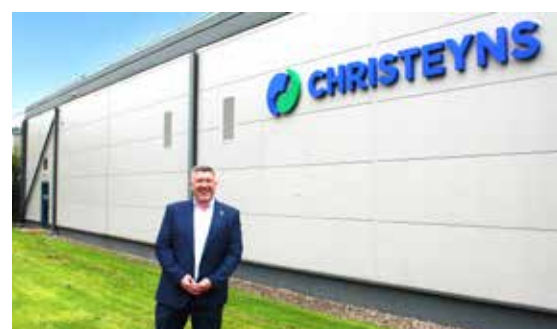
Site photo Christeyns Food Hygiene facility at Winwick Quay, Warrington
