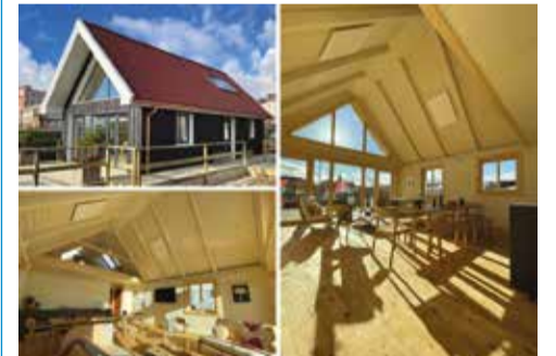
The COP 26 House co-sponsored by Ecomerchant and built for the Glasgow COP is an all-timber construction with no steel, concrete or plastics used in its construction. Insulation is Steico wood fibre, heating by Herschel infrared panels. The COP26 House beats the RIBA 2030 Challenge carbon target by a substantial 22%
