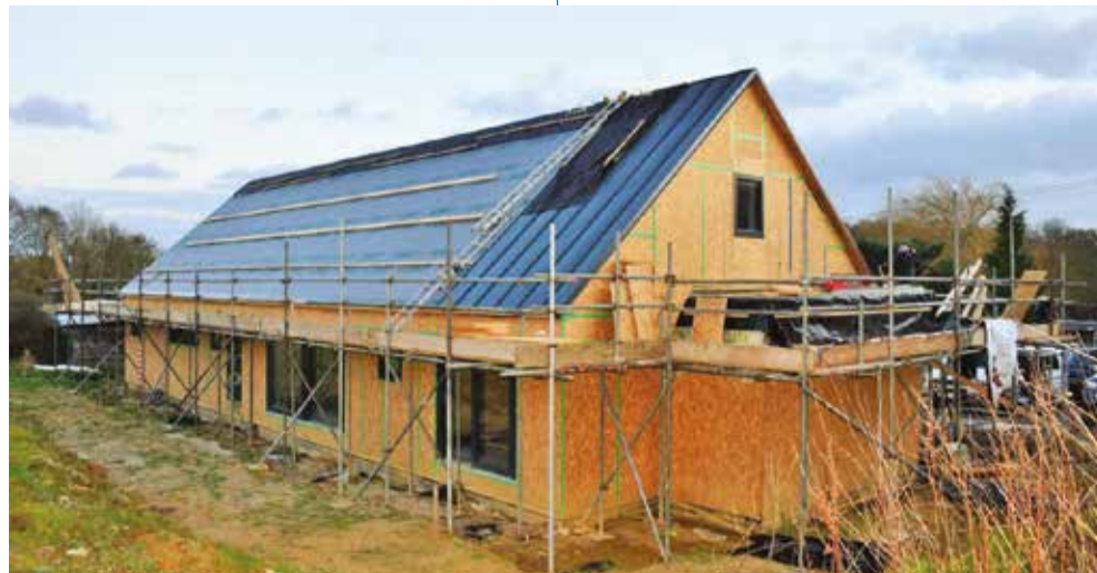
Family house built with naturally insulated passive panels (NIPPs) constructed to passive levels of airtightness and energy efficiency, the complete construction is made using natural and sustainable materials. Image courtesy of Kithurst Builders.
