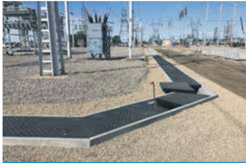
Custom Fibrelite covers installed in precast concrete manufacturer Trenwa's troughs at major US sub-station
