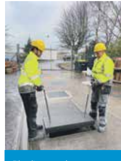
Fibrelite trough covers are designed to be safely and easily removed by two people
