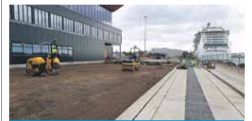
F900 (90-tonne) load rated GRP Fibrelite trench covers in precast concrete troughs/trenches at a cruise ship terminal
