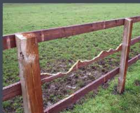
Incorrect treated timber fencing used for horses.
