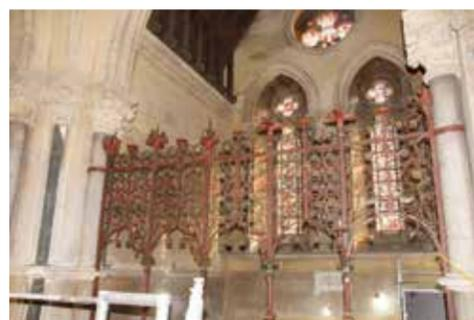
had become dirty, with some losses due to localised iron corrosion which could possibly be linked to condensation during cold weather periods. The client instructed HMCC to carry out the conservation recommendations in the original report, to clean and stabilise the screens, altar rail and wall lights. This was done as
