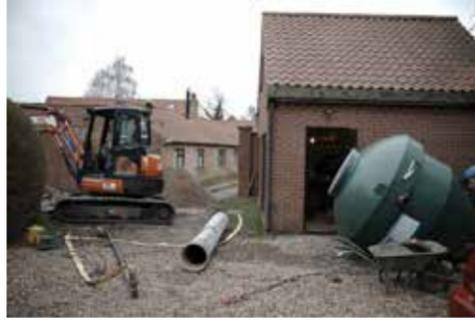
Installation inside your existing septic tank also means that the ConSept cannot be seen or heard, and the air blower remains outside the tank for easy maintenance. The equipment also has low maintenance costs, requiring servicing just once a year and desludging and emptying
