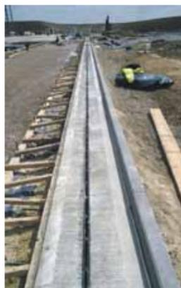
the 200, 300 and 680 sizes were installed in a step fall arrangement providing an enhanced water volume for these runs of 366,324 litres per metre (l/m). All the sizes supplied had fixed ductile iron, 14mm open slot inlets finished with KTL, a rust resistant coating. All 1229 metres of RECYFIX® HICAP® channel installed complied with loading category Class F900 (900kN).
