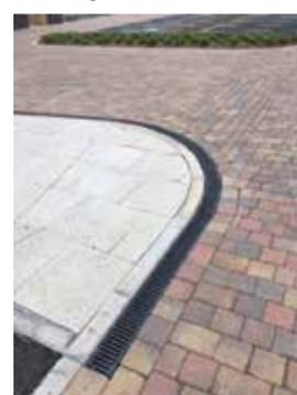
is made of tough, virtually unbreakable polypropylene (PP) formulated to be very resistant to daily temperature fluctuations from frost conditions to strong sunlight, including the Ultra Violet (UV) spectrum. PP is naturally resistant to de-icing salt. Complying with
