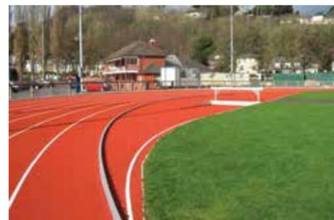
aluminium finishing edges were installed around the perimeter of the IAAF, 400 metre track and along its straight. A steeple chase water jump kit was also installed plus Hauraton SPORTFIX<sup>®</sup> Sand traps and soft edging were installed around the long jump pit.
