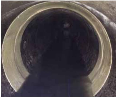
five point repairs, also known as patch liners, to rectify defects and strengthen the pipe so it can withstand high water flow rates, especially during high tides.
