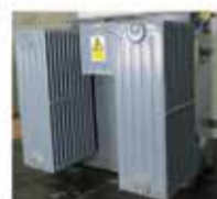
Step Up / Down Transformers
