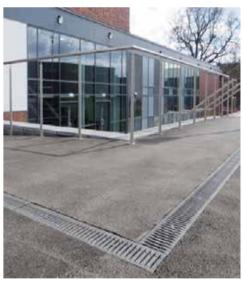
The RECYFIX<sup>®</sup> channel component is made from 100% recycled PE-PP. The six sizes offered are 160mm wide and range in height from 75mm to 201mm with the FIBRETEC<sup>®</sup> grating factory fitted on all models. As the largest unit is only 4.6kg, RECYFIX PRO channelling is easily handle and quickly installed on site.
