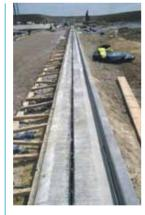
the 200, 300 and 680 sizes were installed in a step fall arrangement providing an enhanced water volume for these runs of 366,324 litres per metre (I/m). All the sizes supplied had fixed ductile iron. 14mm open slot inlets finished with KTL, a rust resistant coating. All 1229 metres of RECYFIX® HICAP® channel installed
