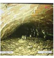
specialists are also working on the project to support Lanes and identify the best way to clear the concrete which is stuck fast to the walls of the 1.2-metre-high bricklined Victorian sewer.
